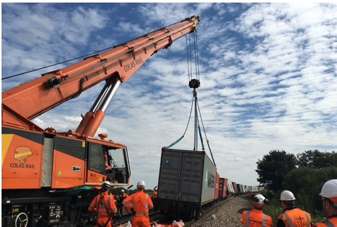
Fig. 1. A crane's lifting the derailed wagons in Cambridgeshire [12]
